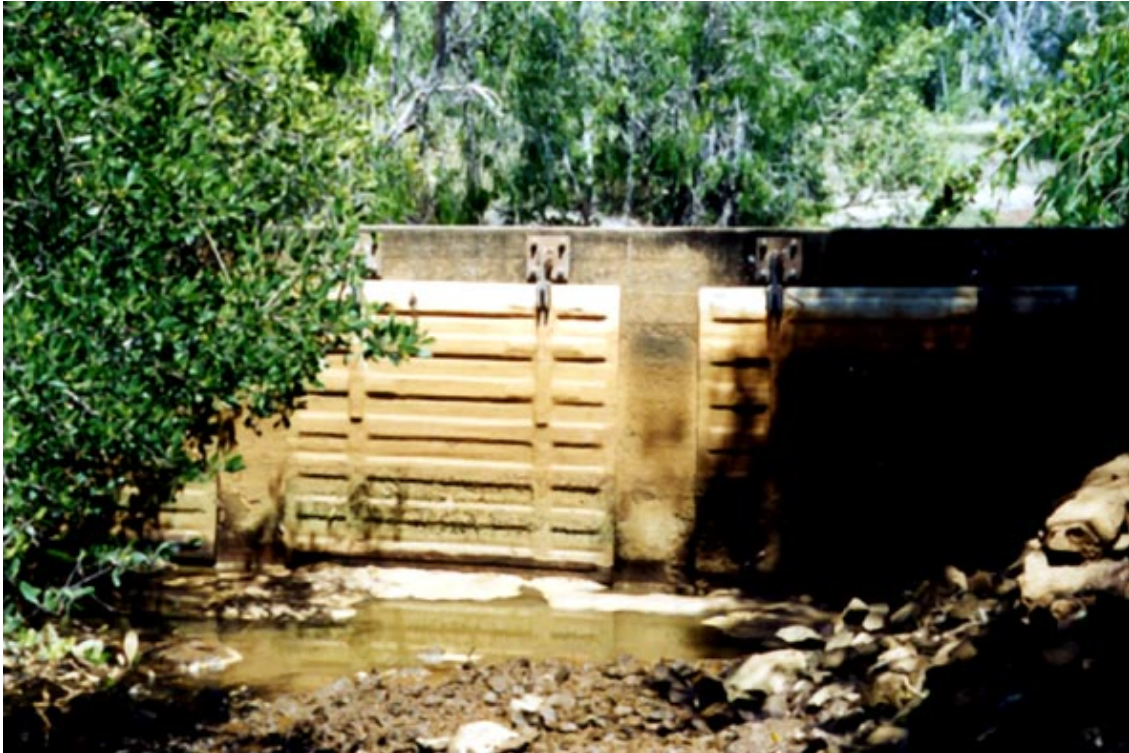
Figure 29: Floodgates preventing tidal intrusion on Mandam wetlands
