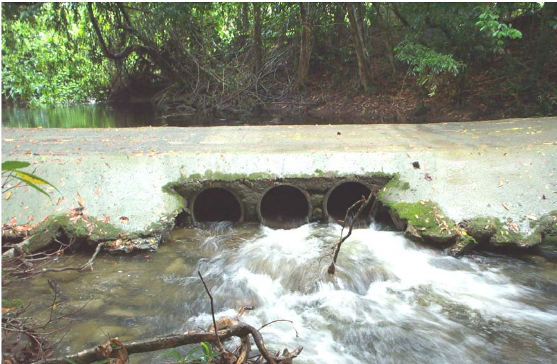
Figure 7: Culvert with high velocity water flow that reduces fish migration on a Saltwater Creek tributary
