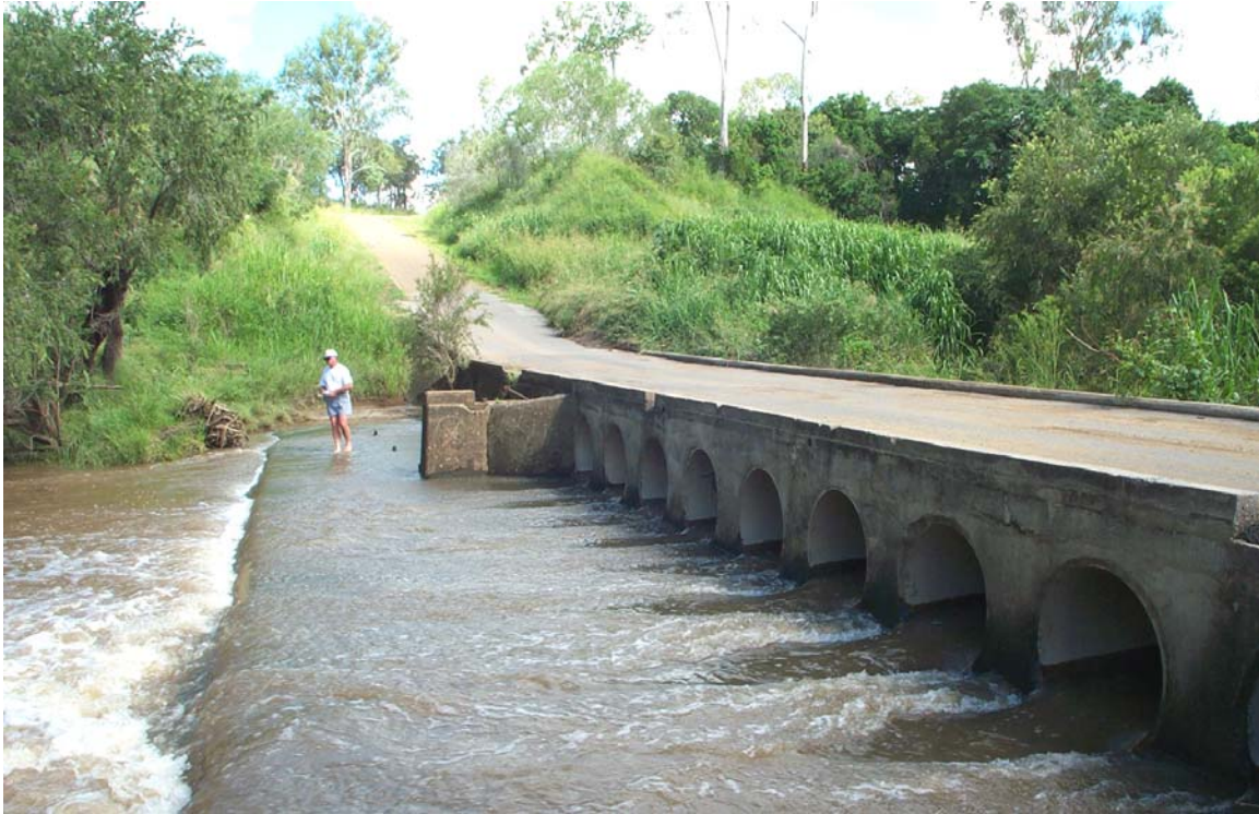
Figure 66: The causeway on Raglan Creek during a flow event indicating obstacles to fish migration
