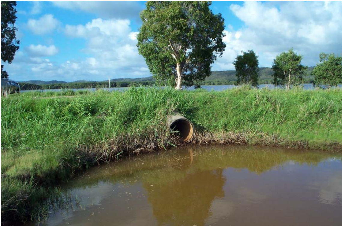
Figure 53: Pipe under the roadway and levee bank separating brackish water in foreground from freshwater wetlands in background (juvenile barramundi and other species have been recorded below the pipe)
