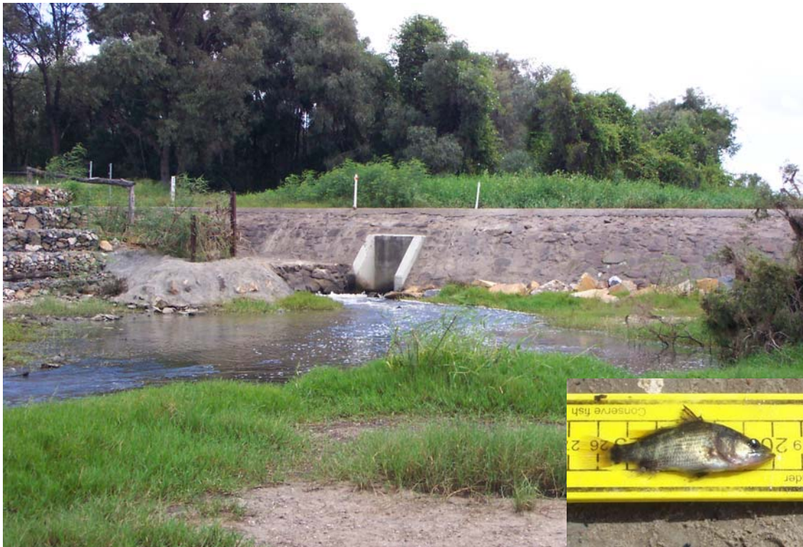
Figure 63: Bajool weir showing the overflow pipe on the downstream side Inset: Juvenile barramundi of 67mm caught below the weir
