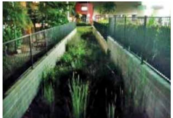
Top quality: bio-retention system located in Airlie Beach
