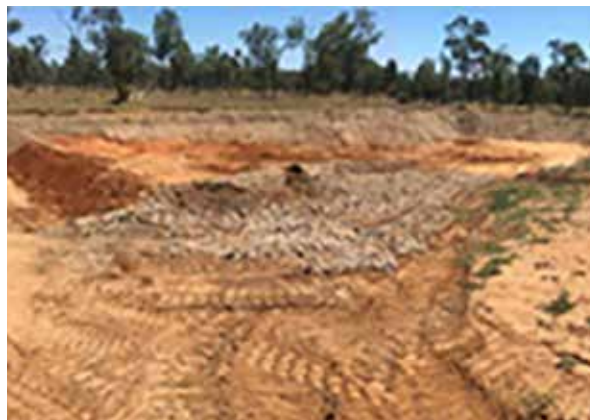
Work in progress: Detention Basin 5 completed and waiting to be hydro-mulched
