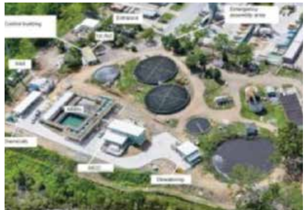
Upgraded: aerial layout of the Cannonvale Sewage Treatment Plant
