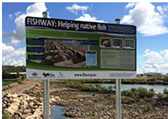
Creating connections: the new fishway passage is located at Lake Callemondah, Gladstone
