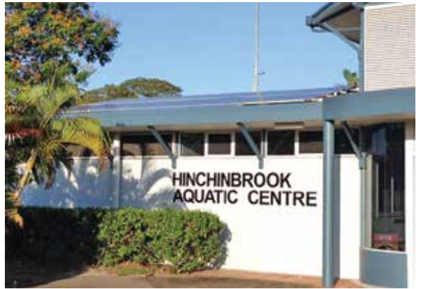
Sustainable power: council's pilot solar project takes off at the Hinchinbrook Aquatic Centre
