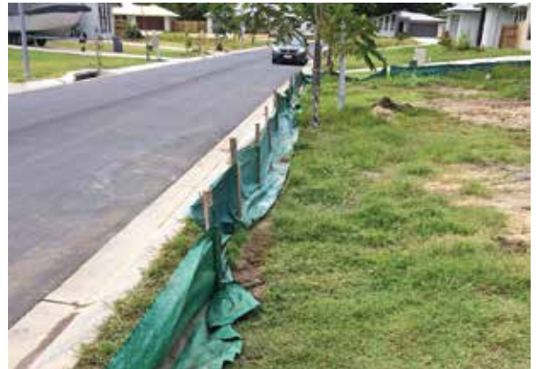
Strategic controls: a sediment fence erected at a development site
