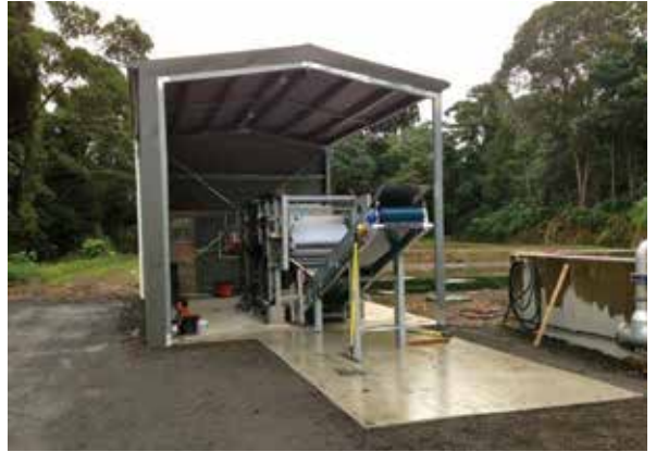
Upgraded: Kuranda Sewage Treatment Plant's new sludge belt press plant
