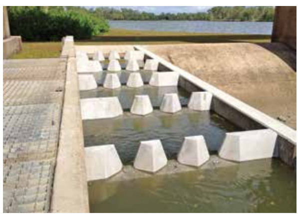
Fast flow: the new fish ladder at the Fitzroy River Barrage has increased passage to 400 fish per minute
