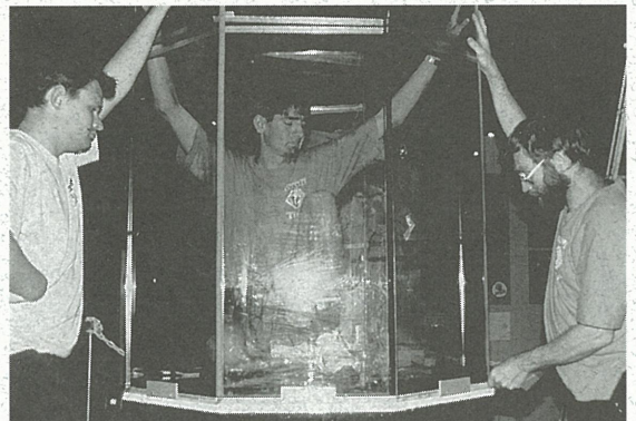
Refitting glass to octagonal tanks, GBR Aquarium. Photo: Glenn Shield
