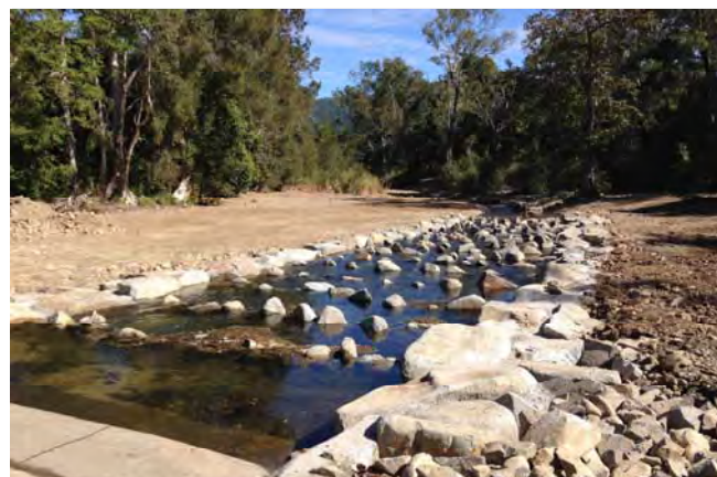
A rock ramp fishway helps fish to move upstream at Porters Rd on the O'Connell River
