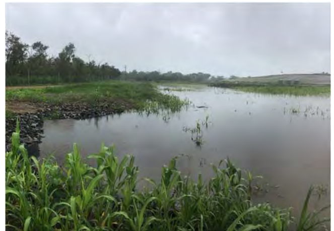
Mareeba landfill surface water management system (landfill in background)
