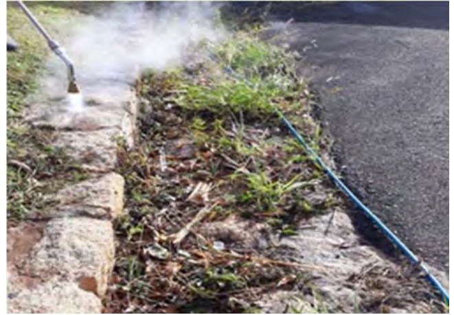
Steam weeding unit removing weeds and grass from the gutters
