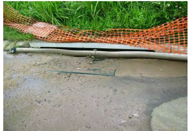
Installation of sediment control in a roadside location
