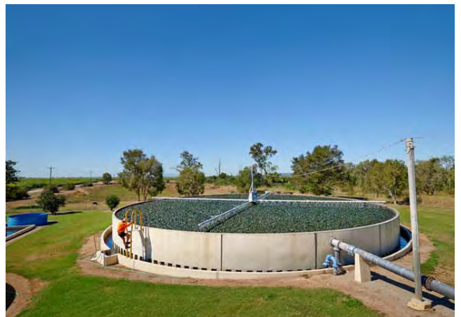
Home Hill waste water treatment plant
