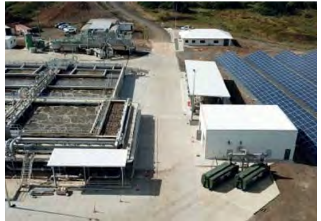
Rubyanna wastewater treatment plant
