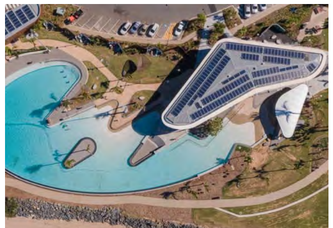
Solar Panels on council's new Foreshore Lagoon building
