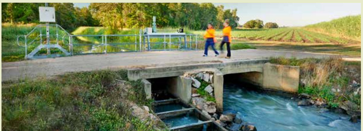
Some structures within waterways provide mechanisms to assist fish to move upstream. © GBRMPA 2016, photographer: Through the Looking Glass Studio
