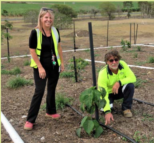
Phytocapping at Qunaba Landfill © Bundaberg Regional Council
