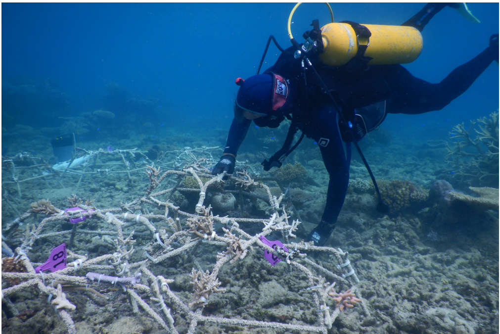
Installation of MARS Reef Stars at Green Island © Commonwealth of Australia (GBRMPA)
