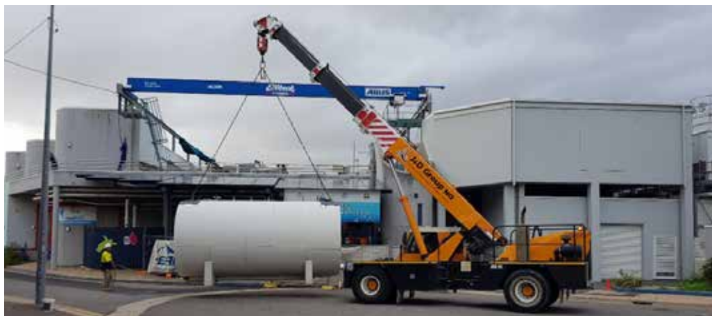
A storage tank for chilled water was removed to enable construction of Reef HQ Aquarium's new access facilities. © Commonwealth of Australia (GBRMPA), Photographer: Jo Hurford
