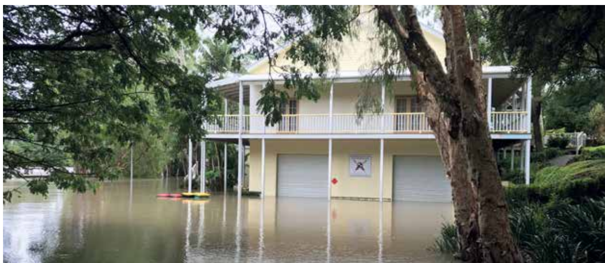
The extreme rainfall event in early 2019 resulted in widespread flooding, inundating homes, businesses and local sports clubs, such as the Townsville and James Cook University Rowing Club. © Chloe Schauble
