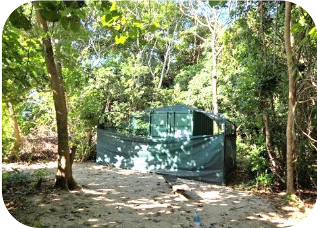
Container installation on Bajigal.
