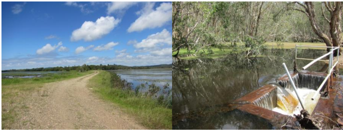
Figure 2: Bund wall (left) and fish barrier (right) in the upper catchment area adjacent to the Corio Bay Ramsar Wetland (photos courtesy of the Great Barrier Reef Marine Park Authority)
