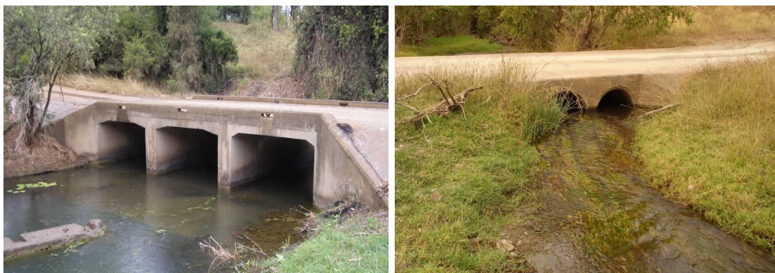
Figure 12: Road crossings that change flow dynamics and act as barriers to fish movement 1
