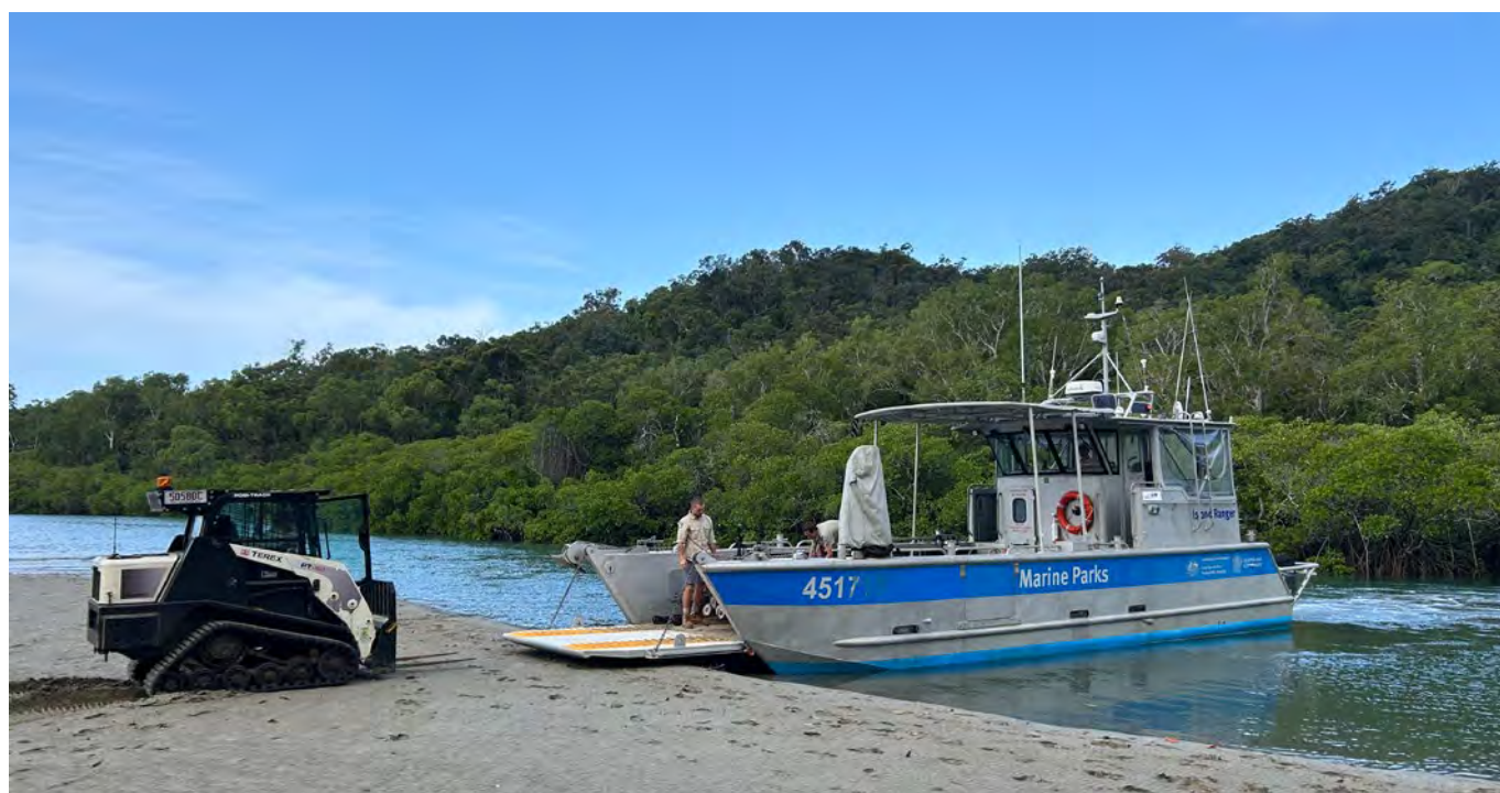
Island Ranger facilitating the works at Munamudanamy (Hinchinbrook Island). © Queensland Government
