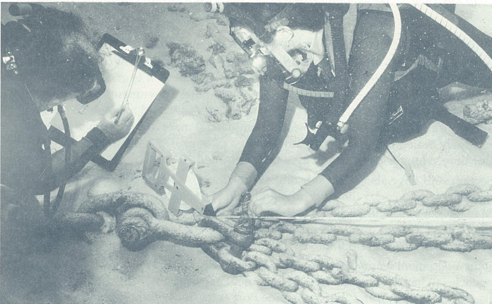
The management of pontoon operations continues to be a high priority. Officers from GBRMPA and QDEH inspect pontoon mooring chains following installation.
