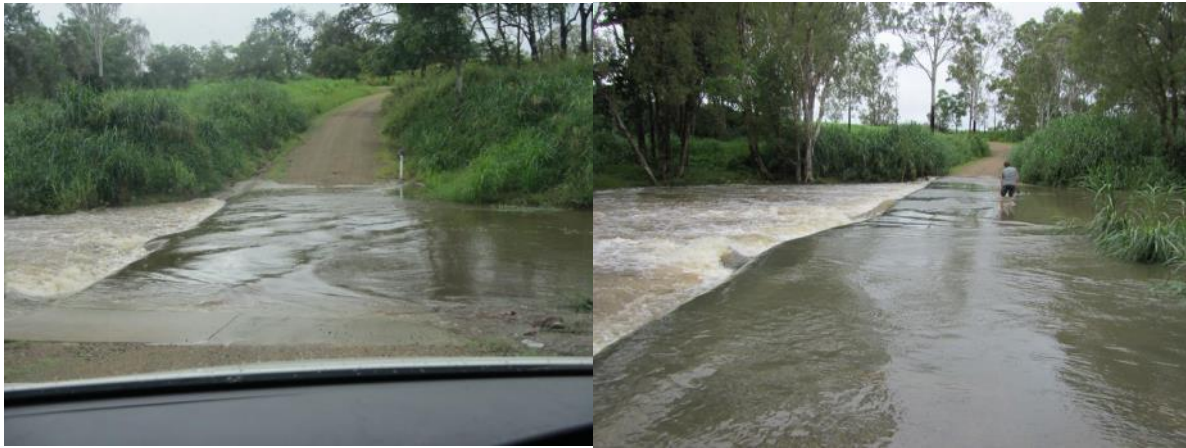
Figure 3.3.3: Examples of road crossings that act as barriers to slow moving native migratory fish
