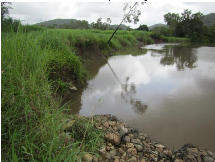
Figure 2.3.13: Jolimont Creek - tributary of Murray Creek
