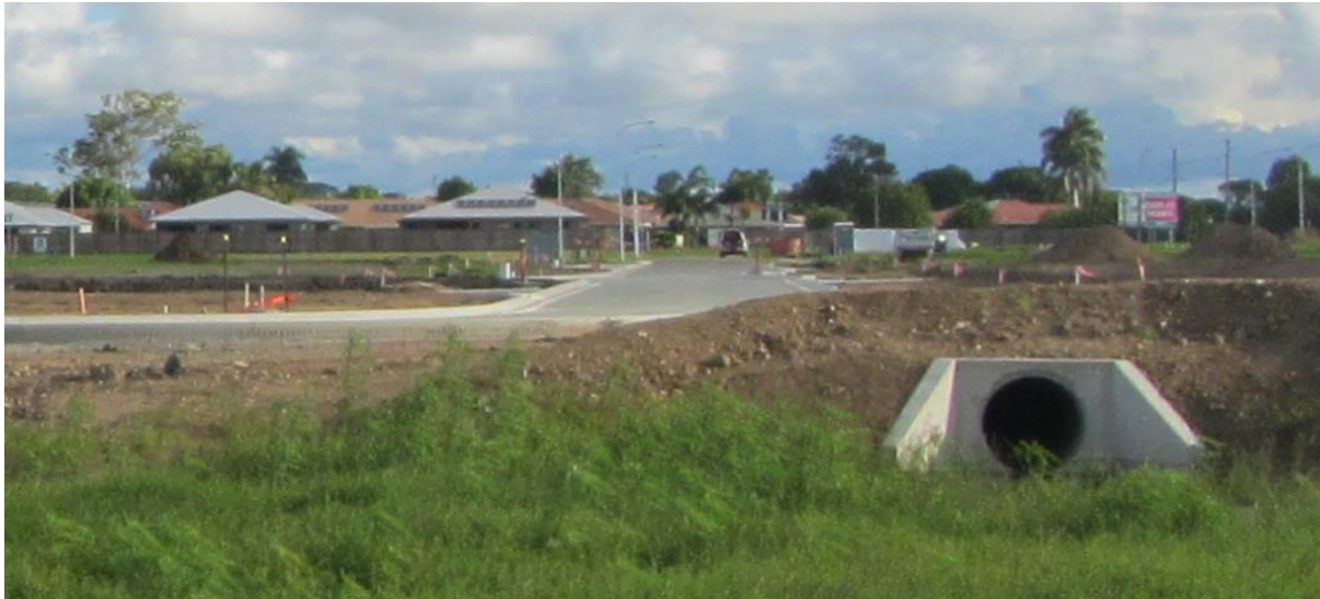
Figure 1: Stormwater management in a new urban development in Mackay
