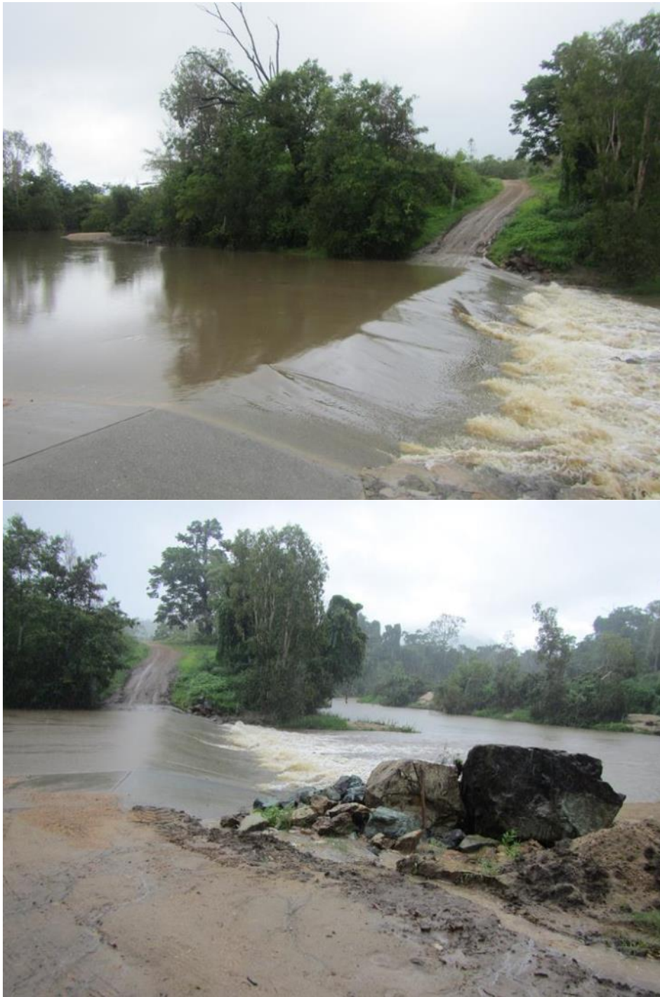
Figure 2.5.3: Road crossing (fish barrier) in the Andromache River during heavy wet season flows. The high rate of flow is impassable by slow moving native fishes
