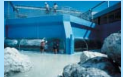
Constructing the coral reef exhibit
