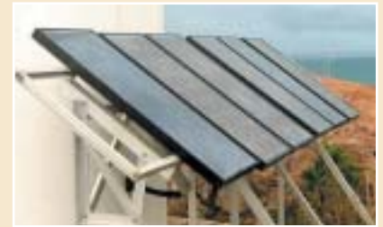
Solar panels have been installed at Low Isles, a Commonwealth island
