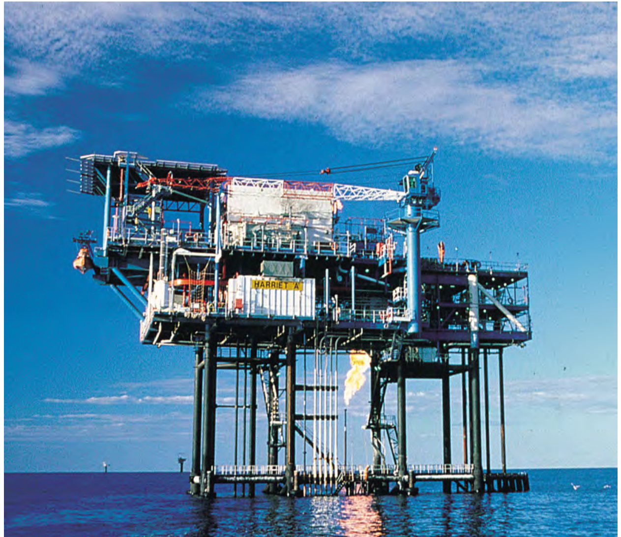
Harriet A gas platform
