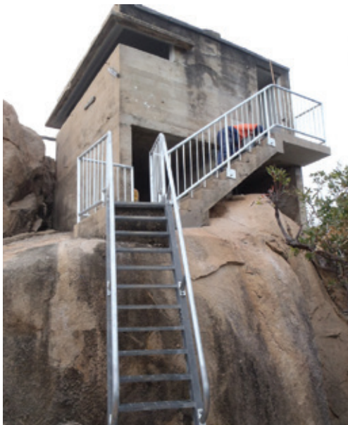
The new railing to the artillery command post at the Magnetic Island forts complex. Photograph courtesy of Queensland Parks and Wildlife Service.
