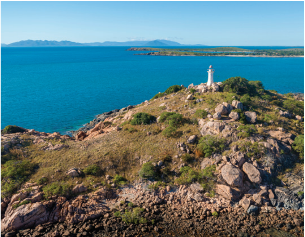
The North Head Lighthouse at the entrance to the Bowen harbour, installed in November 1867
