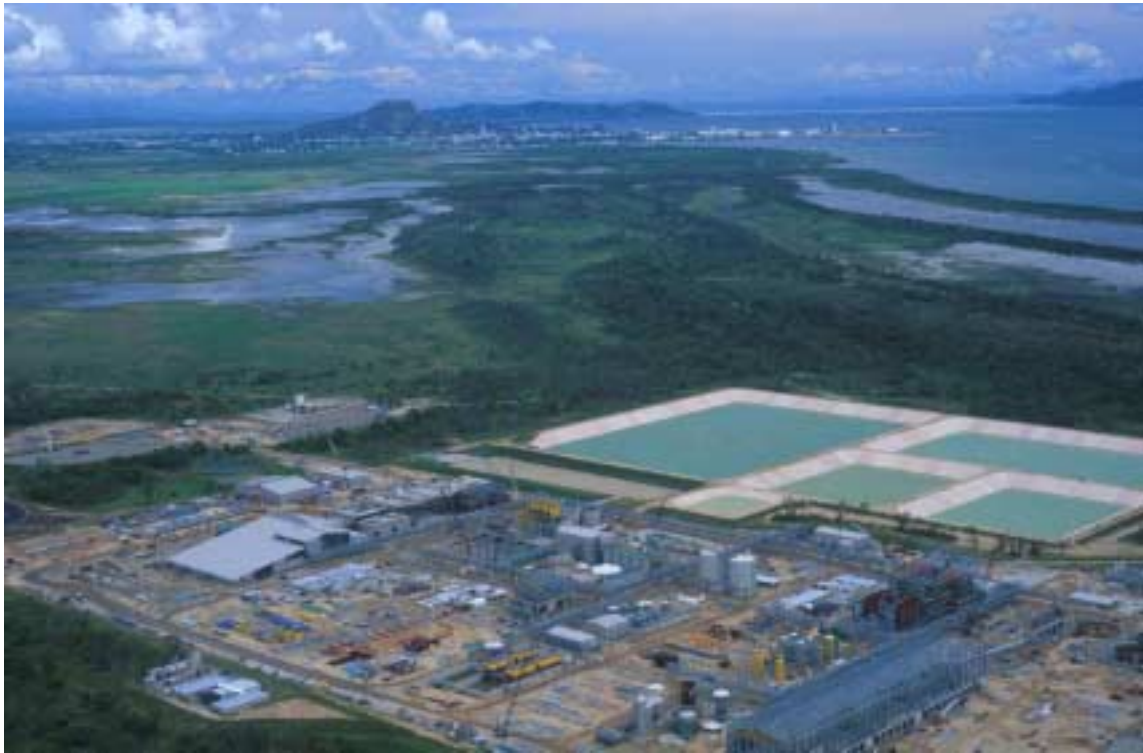
Figure 10. Sun Metals Zinc Refinery, Townsville.
