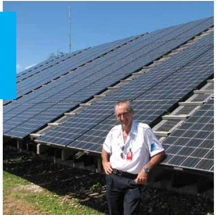
Peter Gash with the hybrid solar power system that powers Lady Elliot Island Eco Resort
