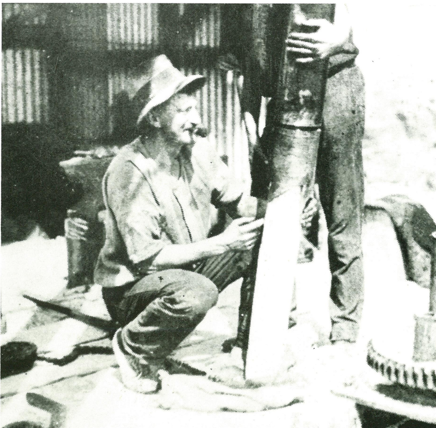
The drilling plant and crew came on loan from the Victorian Mines Department to work on the bore.
