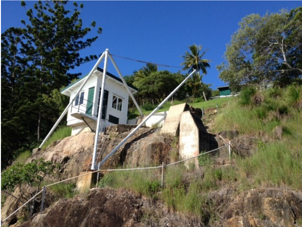
Figure 3 Dent Island's Winch House and Derrick Crane © Commonwealth of Australia (Great Barrier Reef Marine Park Authority)
