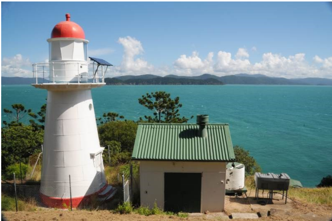
Figure 2 Dent Island Lighthouse © Commonwealth of Australia (Great Barrier Reef Marine Park Authority)
