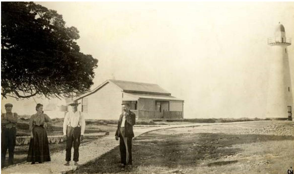
Figure 7 Lady Elliot Lighthouse and cottage, no date, sourced from Australian Maritime Safety Authority
