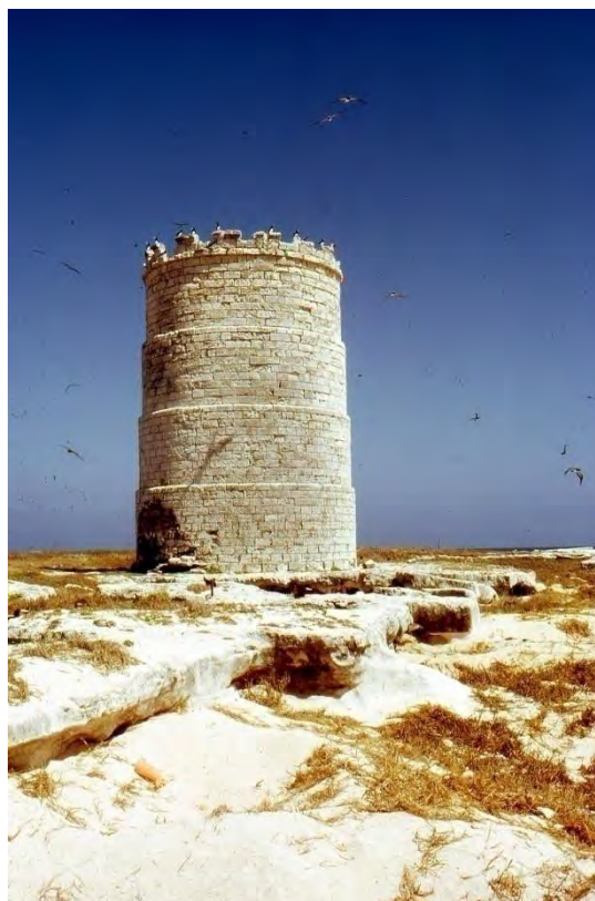
Plate 2: The historic 1844 beacon, constructed from phosphatic cay sandstone © D. Hopley
