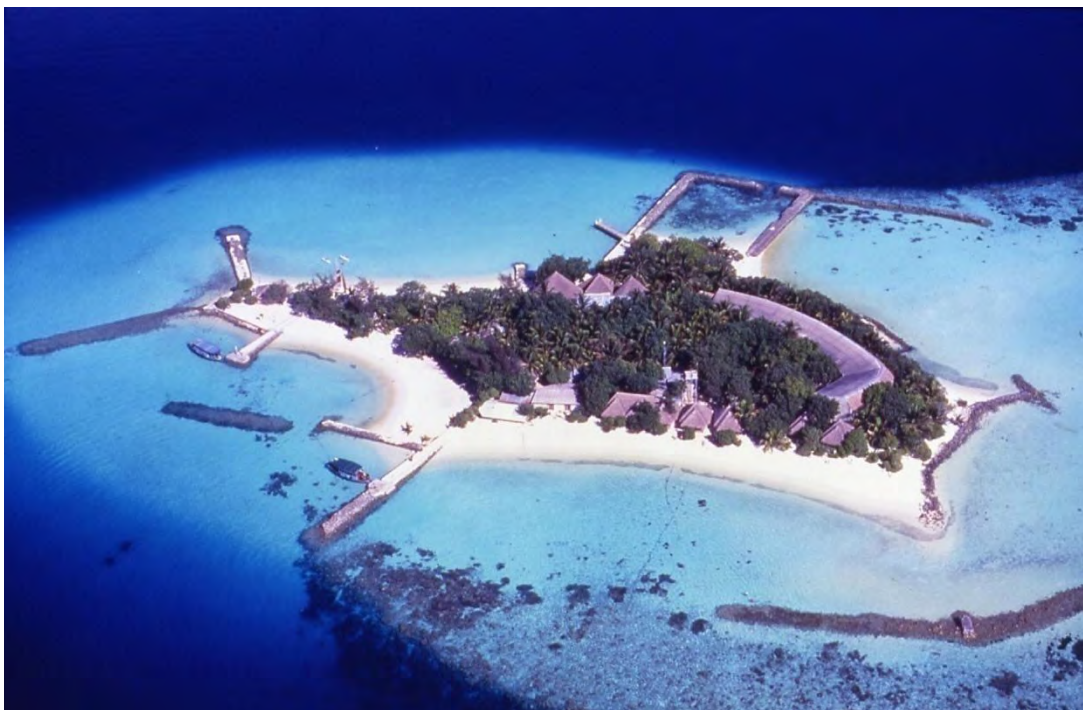
Plate 10: Hard engineering works produce more problems than they solve on coral cays as exemplified by this example of Bolifushi, Maldives. © Mohammed Ali
