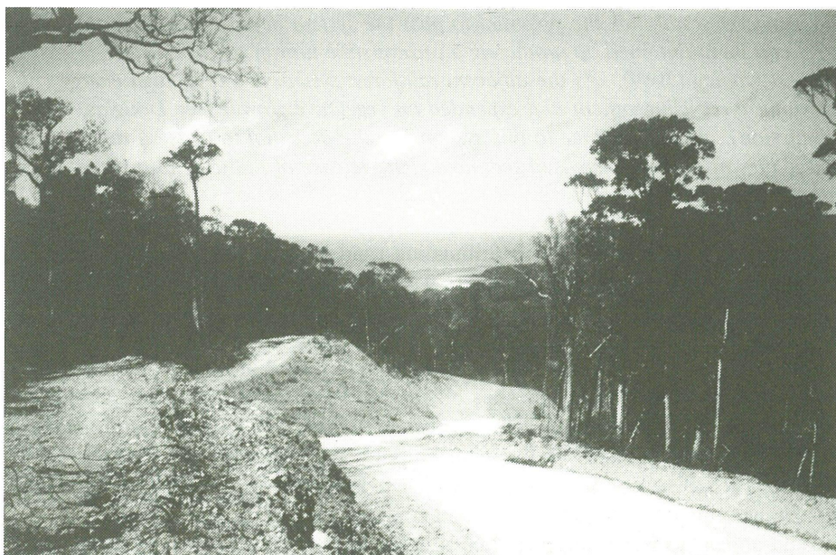
FIGURE 17. Typical road section with steep grades, unstabilised cut and fill sections
