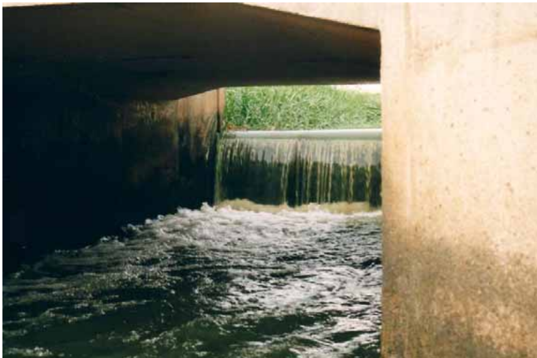
Figure 42: Drop boards on Sheepstation Creek that prevent fish migration except in flooding
