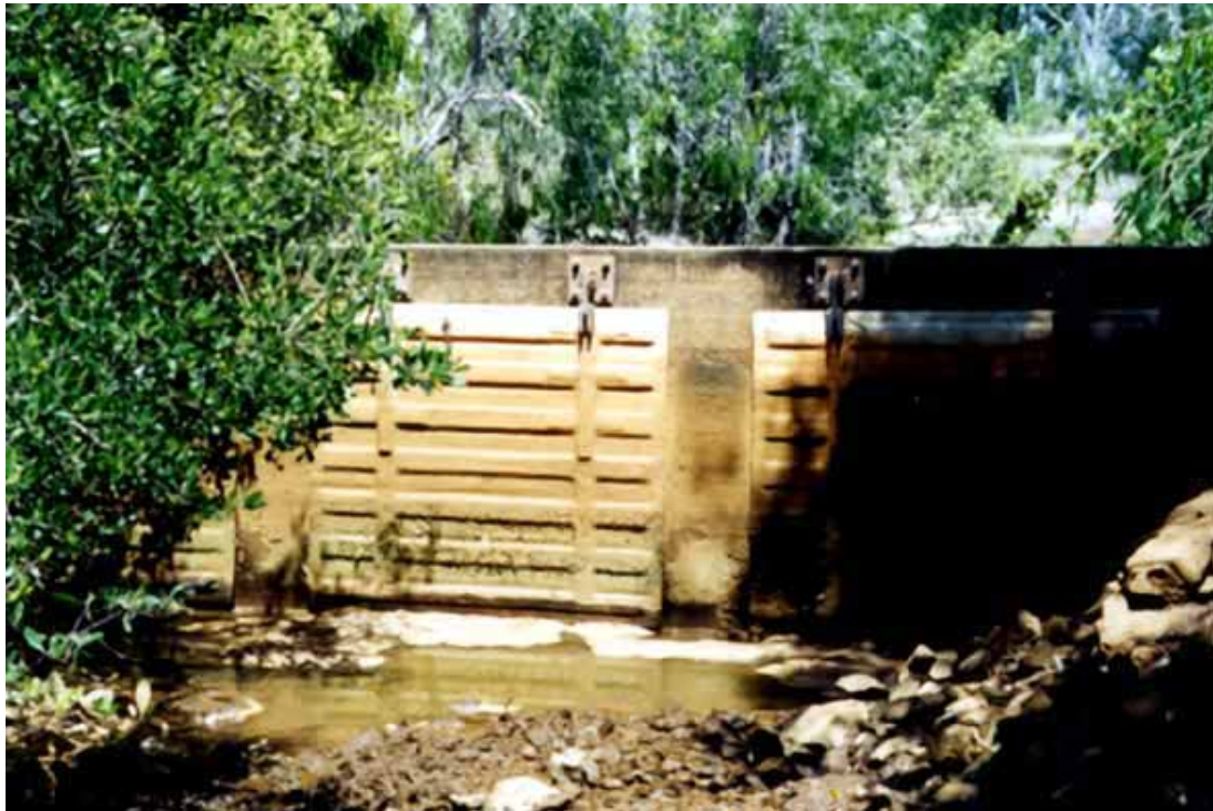
Figure 29: Floodgates preventing tidal intrusion on Mandam wetlands
