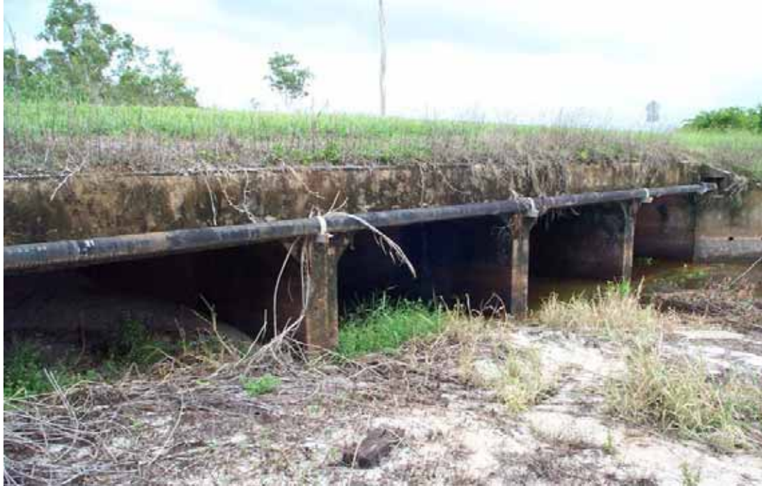
Figure 18: Crossing on Ninds Creek below Bulkuru Swamp showing iron flocculation and concrete corrosion associated with drainage of ASS
