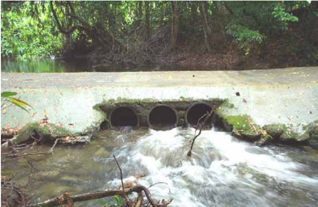
Figure 7: Culvert with high velocity water flow that reduces fish migration on a Saltwater Creek tributary
