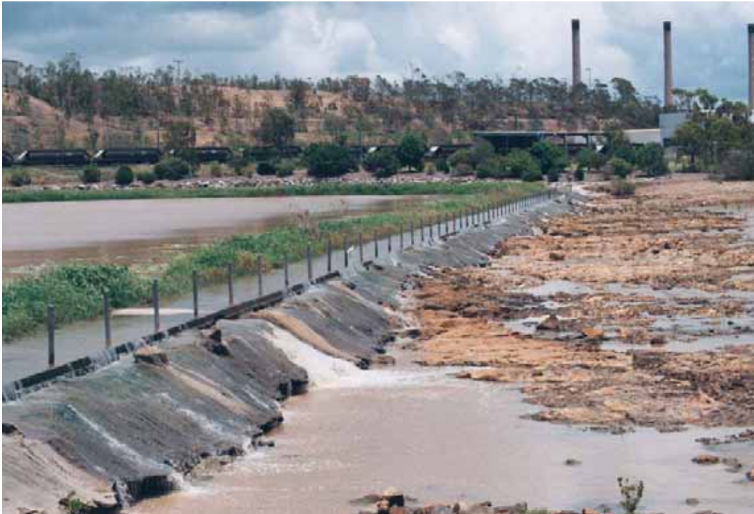
Figure 74: Water overflowing the wall on Lake Callemondah at Gladstone
