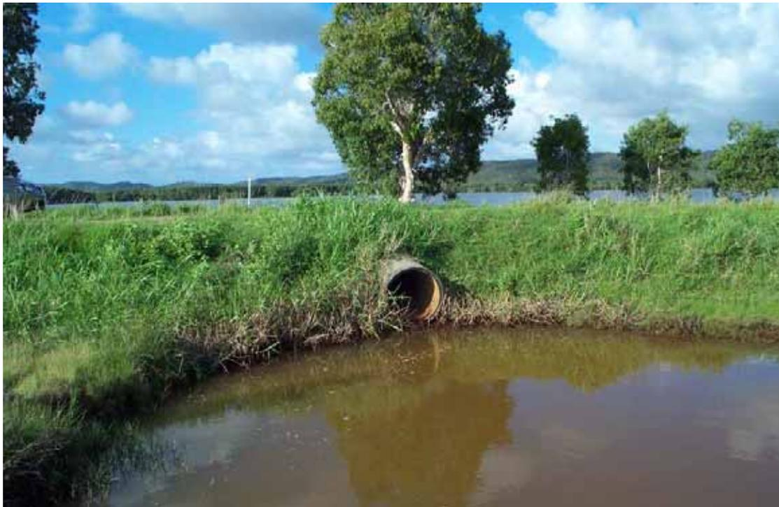
Figure 53: Pipe under the roadway and levee bank separating brackish water in foreground from freshwater wetlands in background (juvenile barramundi and other species have been recorded below the pipe)
