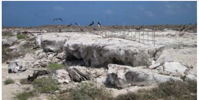
The new fence at Raine Island. Photo courtesy of QPWS
