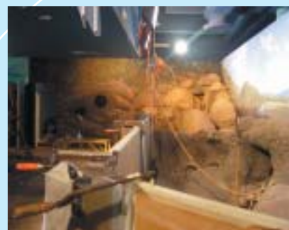
Under construction: The wetlands exhibit begins to take shape
