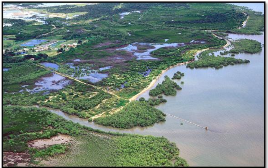
Above: Sewage treatment plant Cleveland Bay, Townsville (circa 1999)
