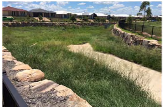
Putting Water Sensitive Urban Design into practice; a bio-swale in Norman Gardens, Rockhampton.
