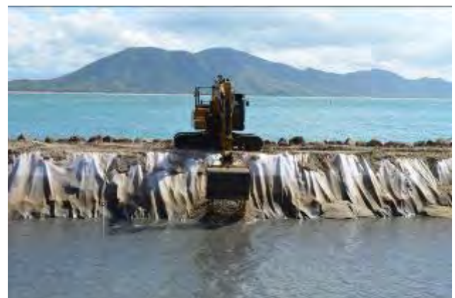
Eco-friendly solution – geofabric will minimise sediment loss from new seawall.
