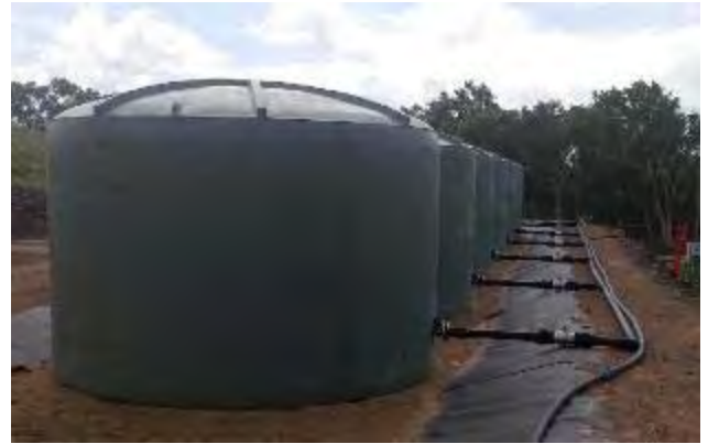
Leachate tanks tackle waste.
