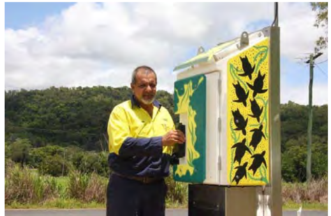
Pump pit control boxes now works of art!
