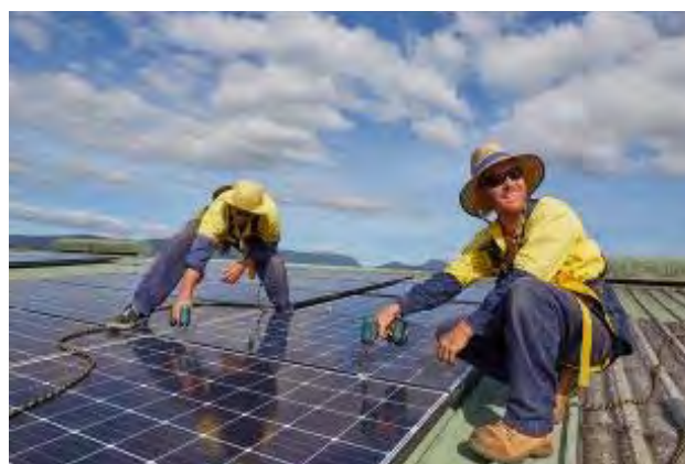
Solar panels light the way to CO 2 target.
