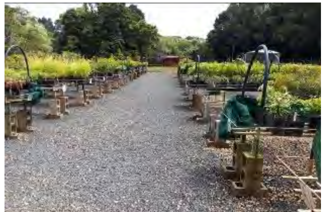
Improved surface drainage at revegetation nursery.
