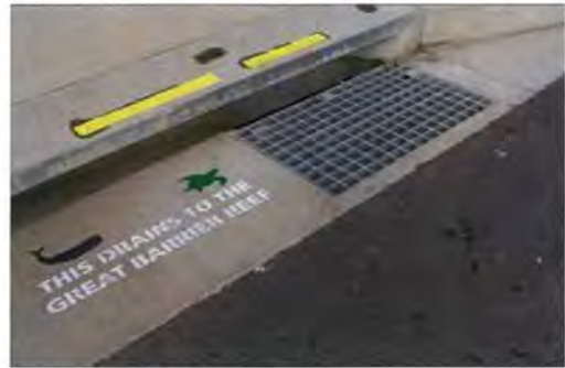
Drain delivers environmental message.
