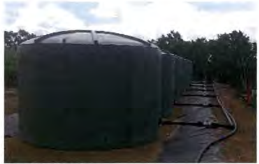
Leachate tanks tackle waste.
