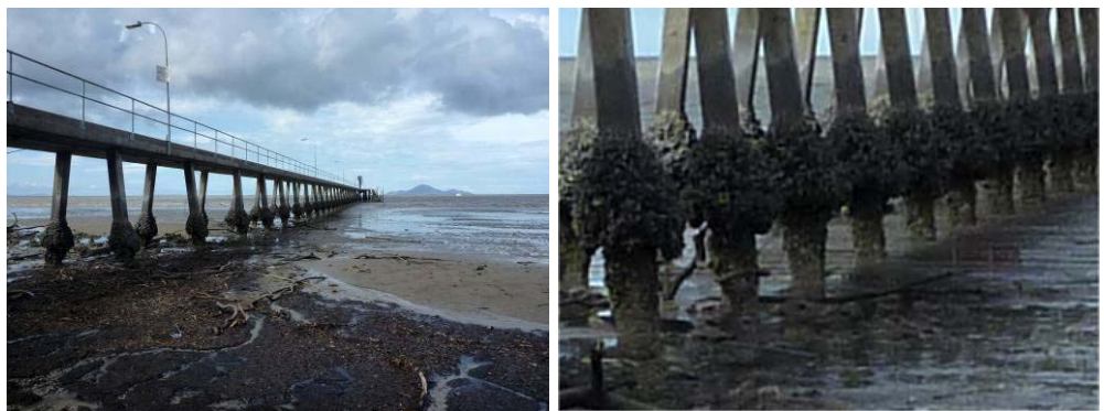
Figure 11. Erosion at Cardwell jetty, 19 February 2011: left) from foreshore, and right) close-up showing height of fouling and clean lower portions of pylons.
