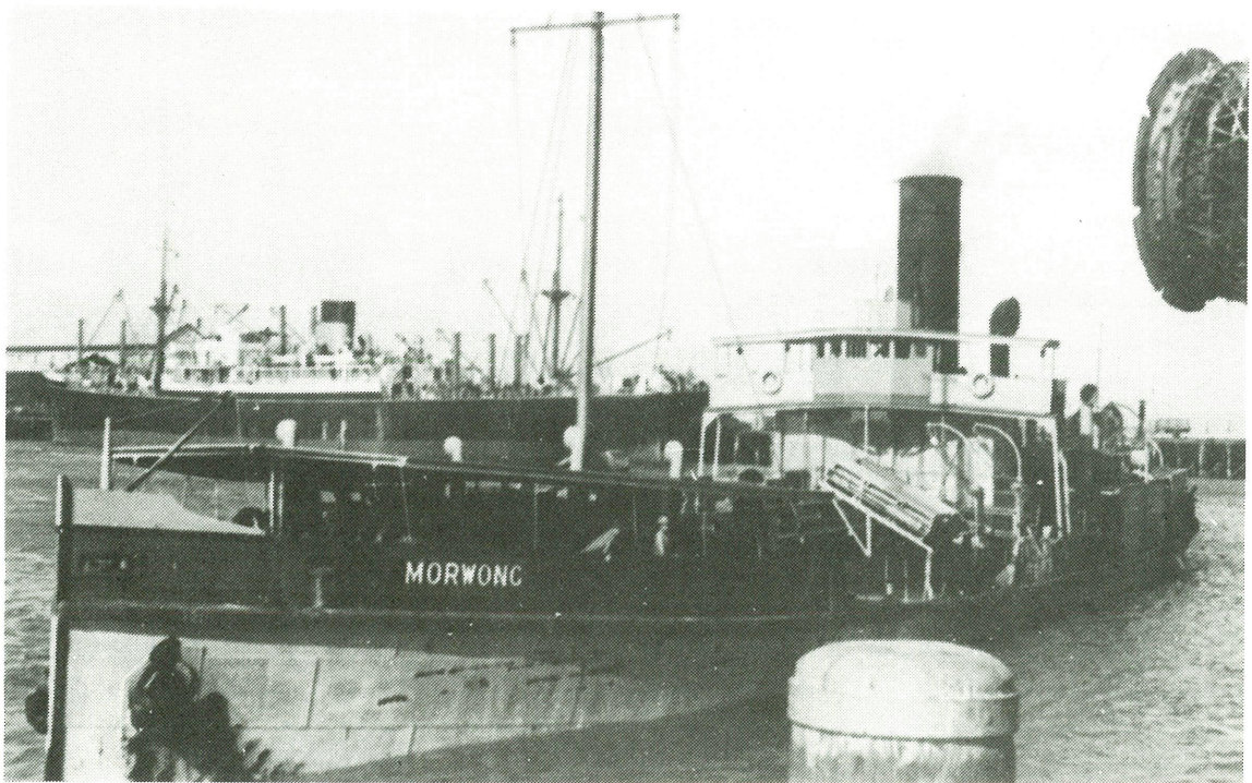
2 Suction Dredge 'Morwong' in October 1946.
